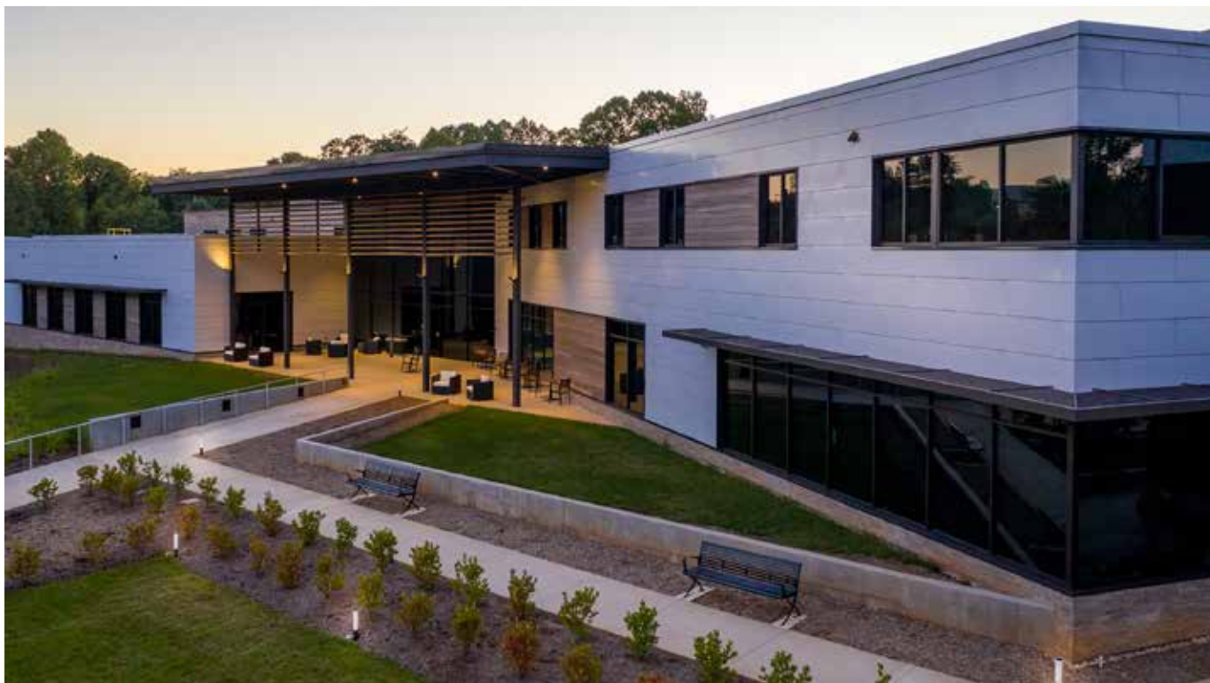
A covered terrace with comfortable seating overlooks green space at the rear of The Center at Belvedere in Charlottesville, Virginia. The lawns can accommodate tents for both Center and rental events. Photo: Gene Runion
